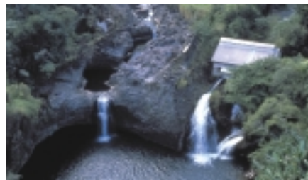
HELCO's Waiiau hydroelectric plant
