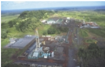
Puna Geothermal Ventures, Big Island
