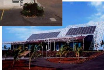
NELHA Gateway Center, 2 x 20 kilowatts
