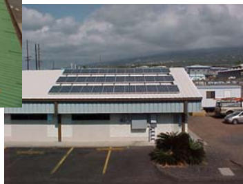
HELCO Kona Baseyard, 5 kilowatts
