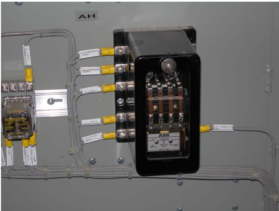
Figure 5: Transmission line AR relay.
