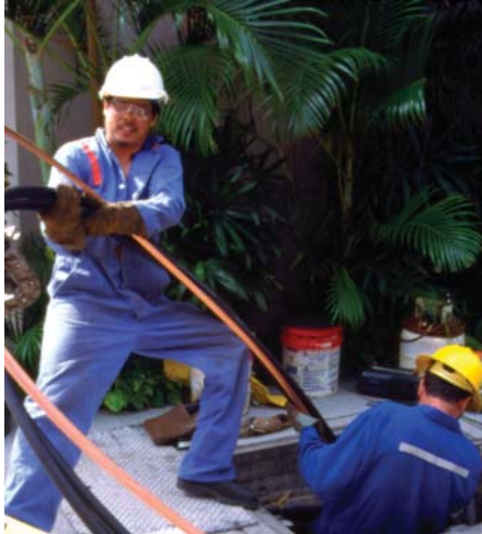
HECO underground crew replaces cables in downtown Honolulu.
