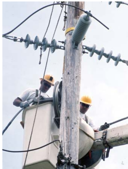
Crews work 24 hours a day to keep the lights on.
