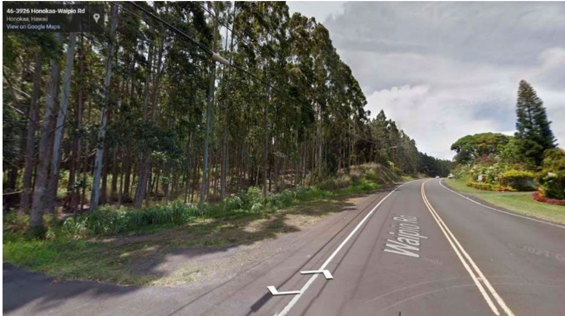
Figure 11 – Honokaa 12kV Circuit 14, Eucalyptus Trees along Waipio Road, Honokaa, Hawaii Island (Google Maps 2022).
