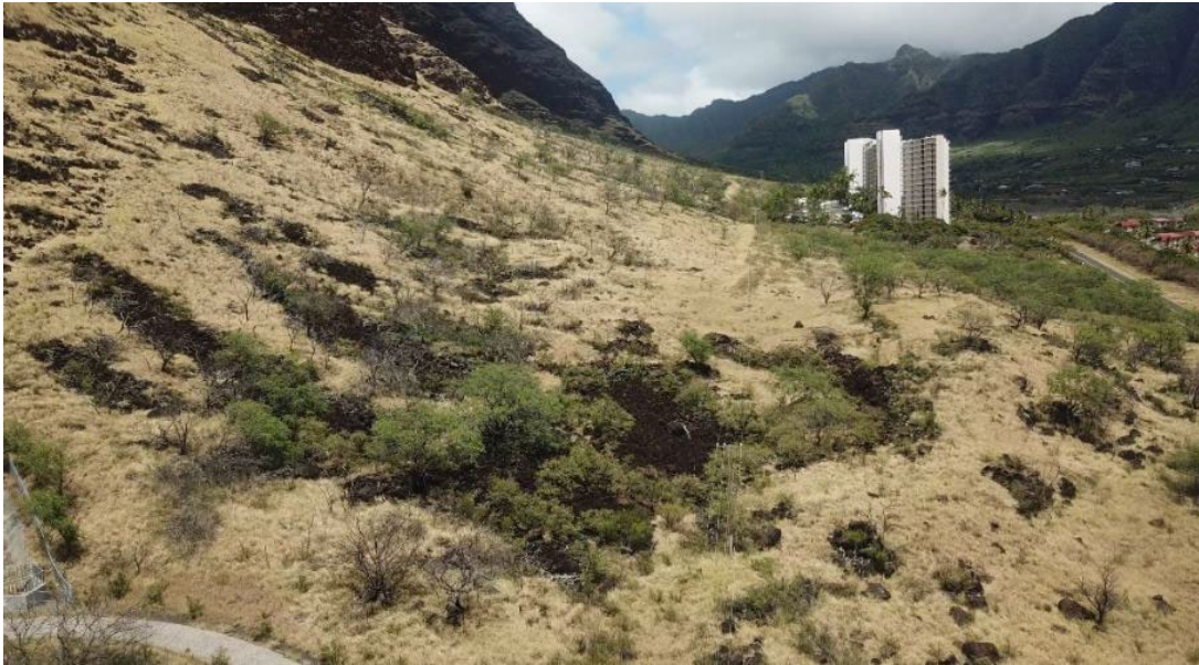
Figure 4 – Makaha Valley 12kV circuit, Makaha Valley, Oahu 2019.
