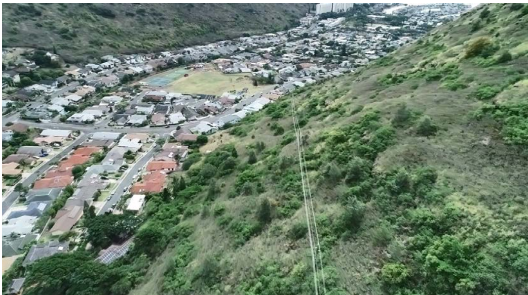
Figure 6 – Koolau-Wailupe #2 46kV Circuit, Hahaione Valley, Oahu.
